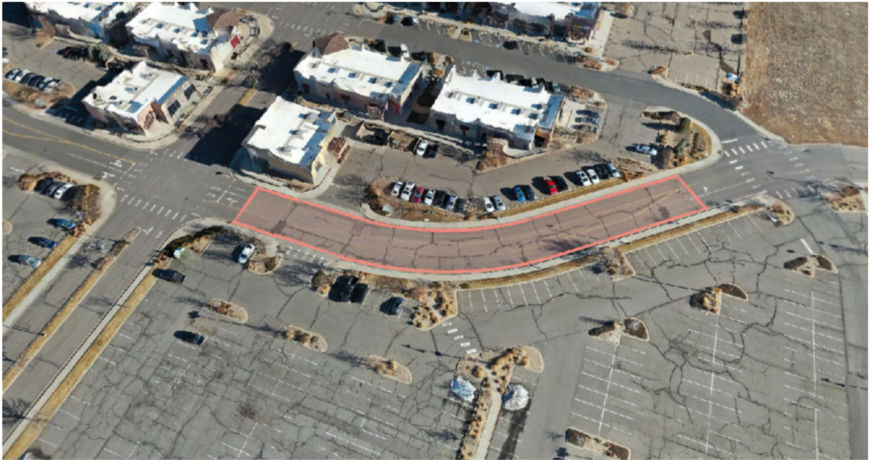
RED AREA - Asphalt Milling & Paving - 2"
